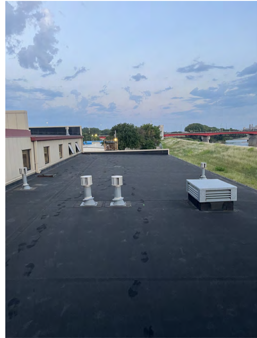
ROOF PHOTO # 5 AREA -2 LOOKING WEST
