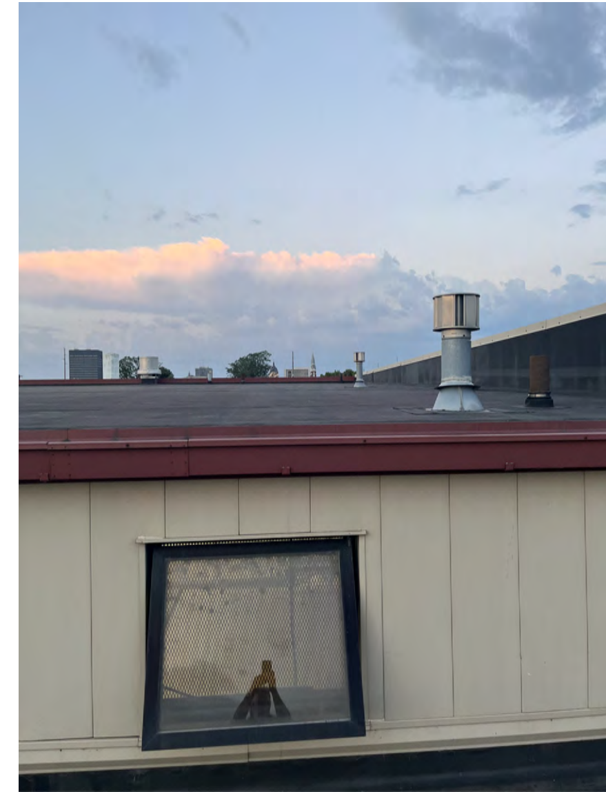
ROOF PHOTO # 7 AREA -3 LOOKING SOUTHWEST
