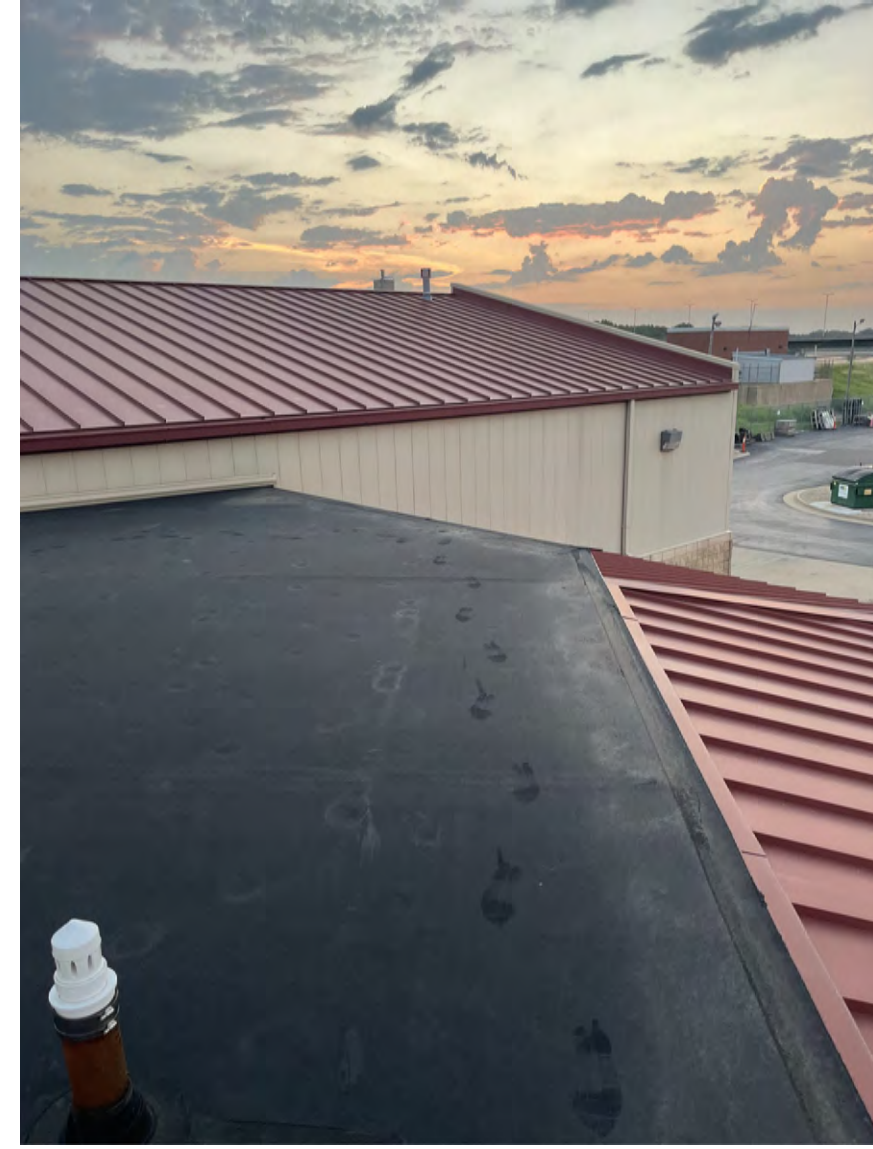
ROOF PHOTO # 10 AREA -4 LOOKING EAST
