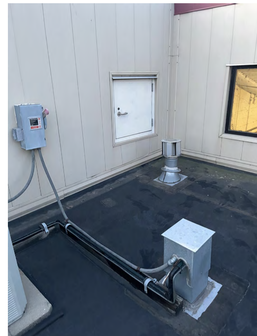
ROOF PHOTO # 3 AREA -1 LOOKING SOUTHEAST
