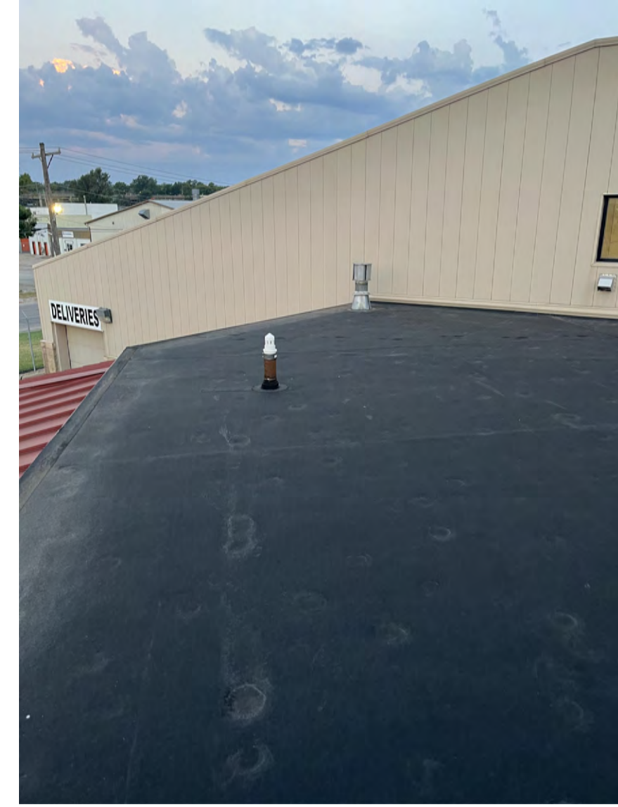
ROOF PHOTO # 11 AREA -4 LOOKING WEST
