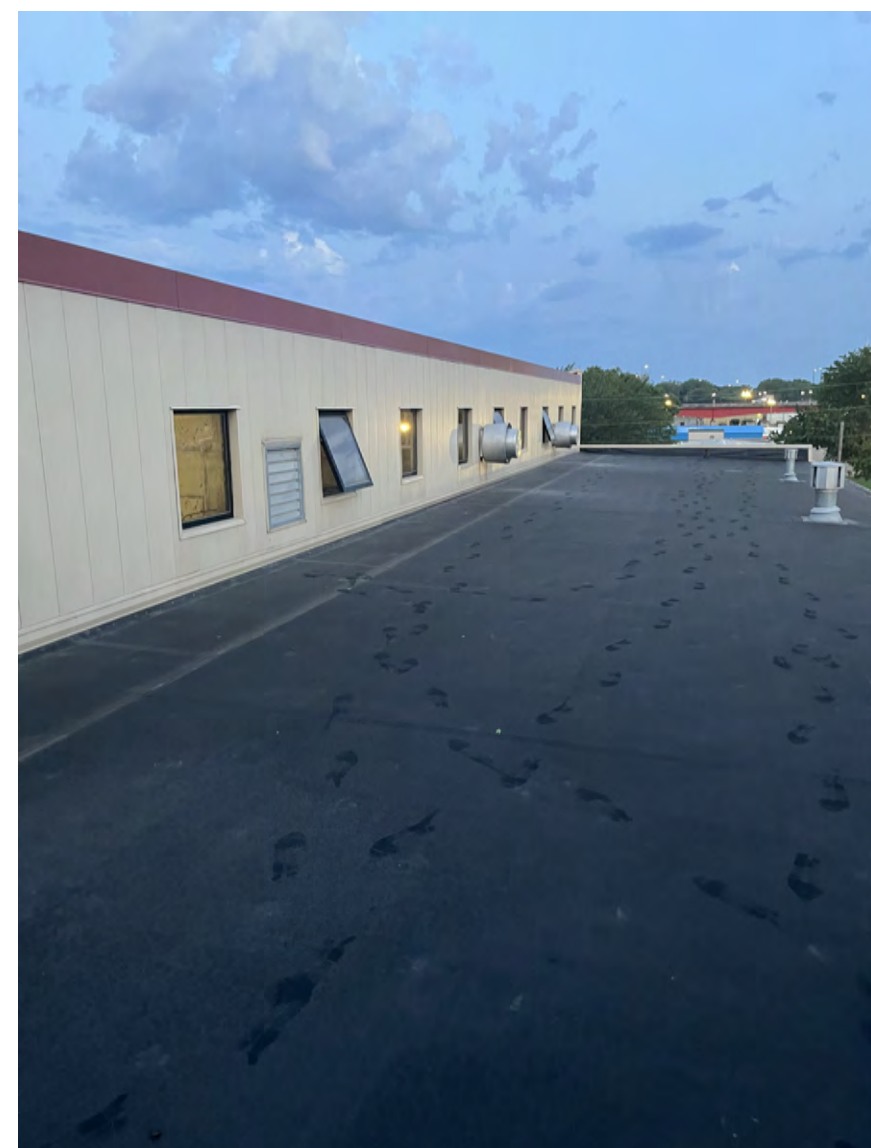
ROOF PHOTO # 1 AREA -1 LOOKING WEST
