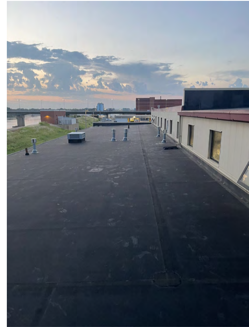
ROOF PHOTO # 4 AREA -2 LOOKING EAST
