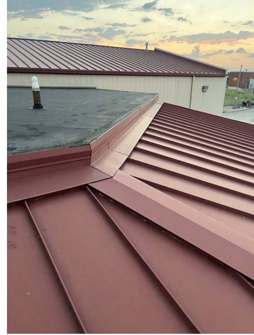
ROOF PHOTO # 8 AREA -4 LOOKING NORTHEAST
