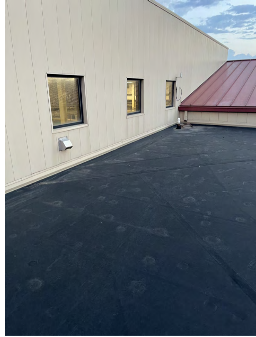
ROOF PHOTO # 9 AREA -4 LOOKING NORTHWEST
