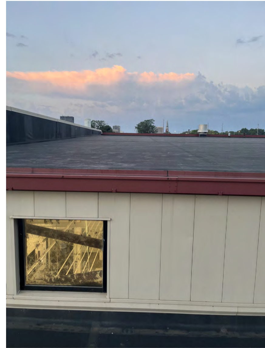
ROOF PHOTO # 6 AREA -3 LOOKING SOUTHEAST
