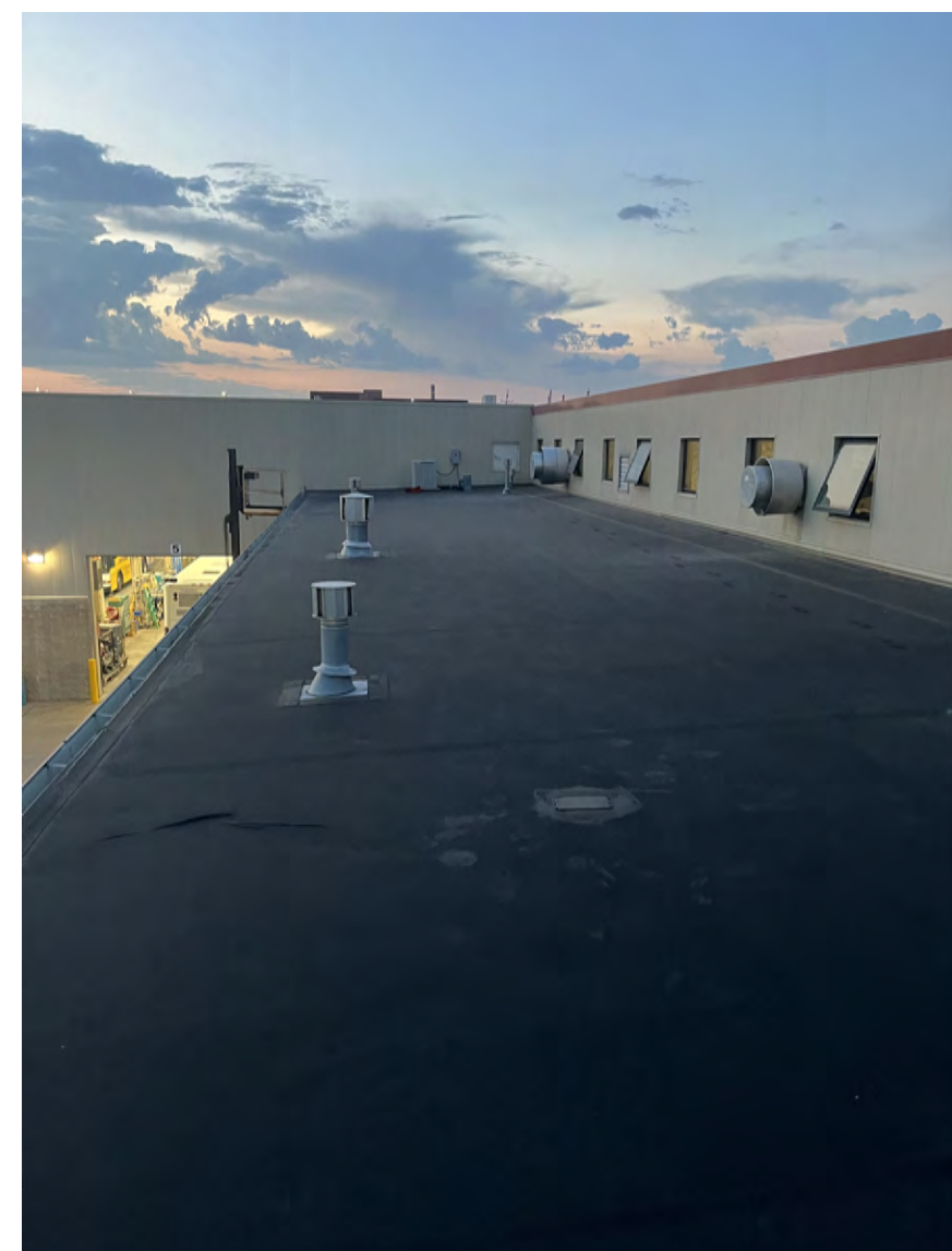
ROOF PHOTO # 2 AREA -1 LOOKING EAST
